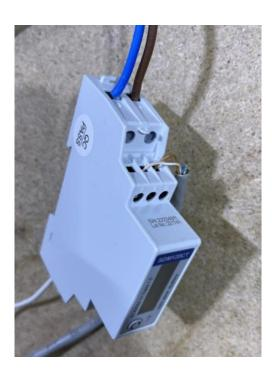
3. Connect the CT coil, black into Port 2 and connect the white into port 1.
