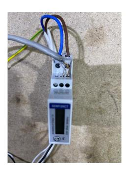
7. On the other end of the CAT-5 cable use a RJ45 connector and slot the brown/white cable into pin 4 and the brown cable into pin 5.
